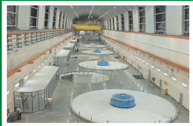
Machine Hall of Tehri HPP (250 x 4 = 1000 MW)
