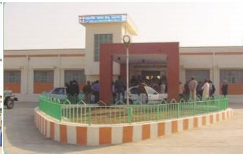
Community Health Centre at Rawatbhata
