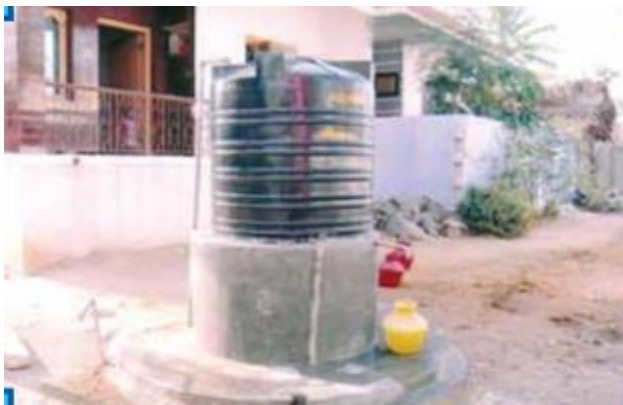
Borewell based watersupply system with Syntex tank
