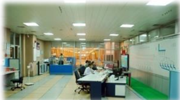
Apprentices in NJHPS Power-House
