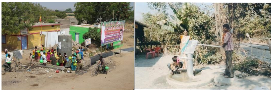
Hand pumps and taps installed by POWERGRID
