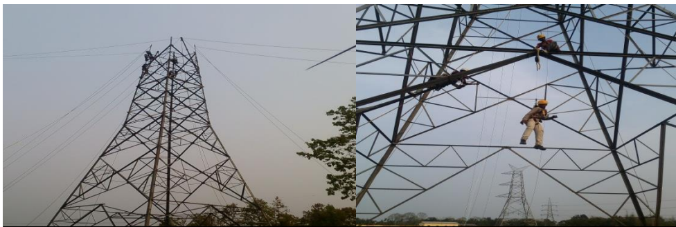
Hands on Training on Transmission Tower Erection and Stringing
