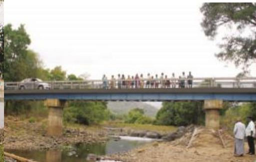
Goyar Bridge near Kaiga
