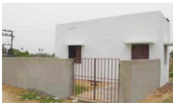
Midday Meal Kitchen constructed at Ayappakkam Govt. School
