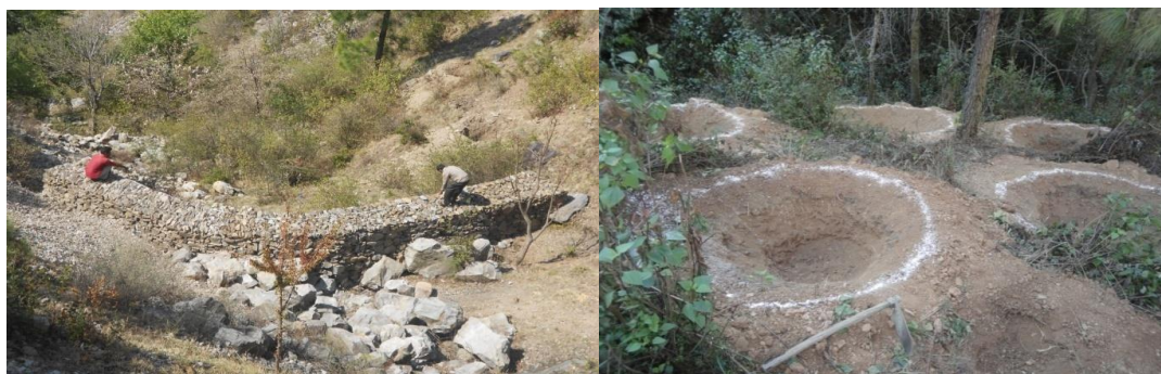
Check dam for water & soil conservation Water recharge pits
