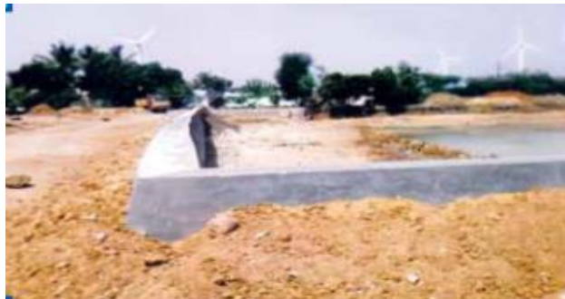
Retaining Wall at TheppakKarunkulam T. Karunkulam
