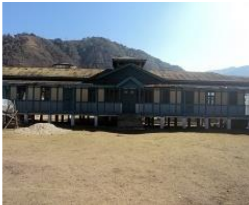
Renovation of Govt Higher Secondary School Building, RHEP, Arunachal Pradesh
